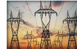
Construction of 500 kV SUTET (450 km) & 500 kV GITET (4 units) for the distribution of hydropower from Kaltara
